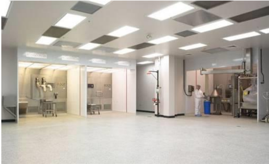
Figure 10-1. Dispensing booths prevent cross-contamination
