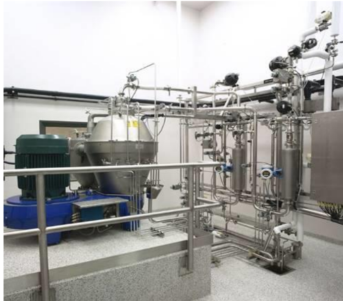
Figure 10-32. A centrifuge, pump, motor and associated piping
