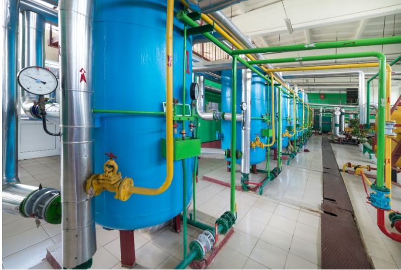
Figure 5.7 Steam Generation System
